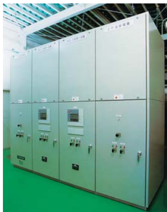
固体绝缘开关柜 要素4.88(SIS/C*1-GIS*2) *1SIS:固体绝缘开关柜(Solid Insulated Switchgear) *2C-GIS:隔离型气体绝缘开关柜(Cubicle type Gas Insulated Switchgear)
